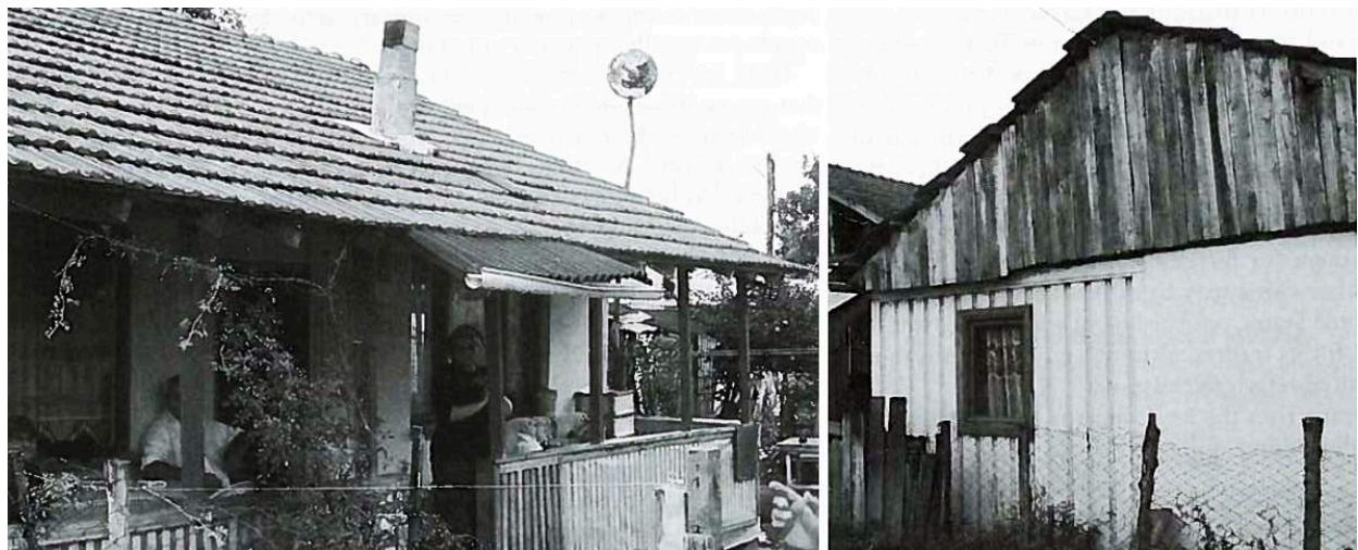
Figure 1.23 - (Left) Front view of the house; (Right) Side view of the housing showing the shipping container, Duzce, Turkey (Source: Book “Rebuilding after disasters” (Lizarralde et al., 2010))
