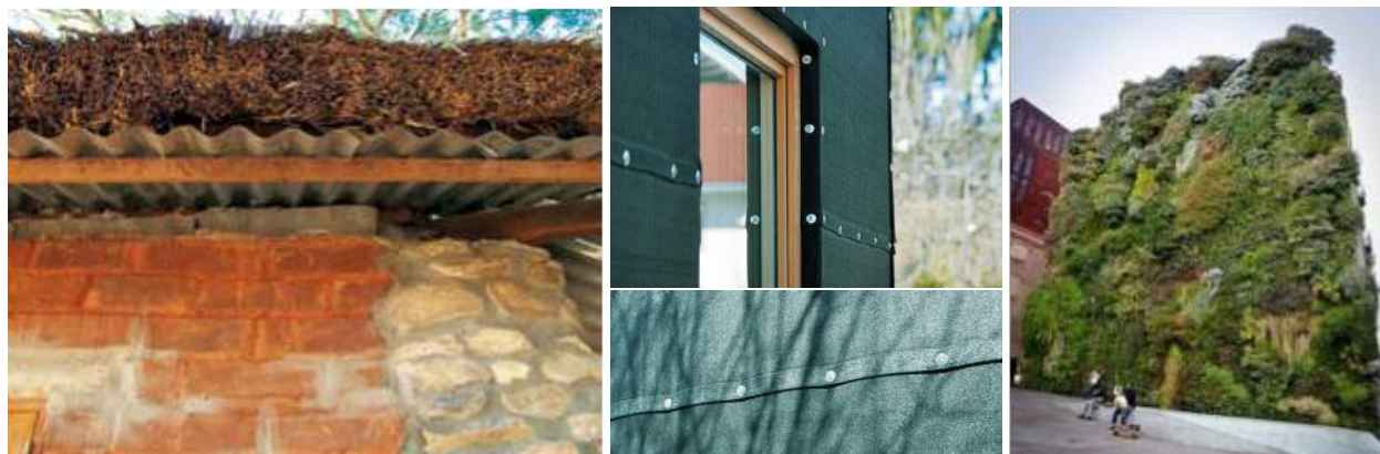
Figure 4.1 – Construction and materials (Left) Constructive system of colm on top of the metal sheets in Angola. Colm adds insulation properties to the impermeability and durability features of the metallic sheet (Source: Manual Boas práticas); (middle) Single-Family House in Feldkirch- Walter Unterrainer : The entire facade, with the exception of the windows, is clad with a matt-black fabric normally used in horticulture http://detail-online.com/inspiration/single-family-house-in-feldkirch-103673.html (Right) Green walls and roofs – living walls in Caixa Forum, Madrid (Source: http://www.pinterest.com/pin/472948398339115095/ )
