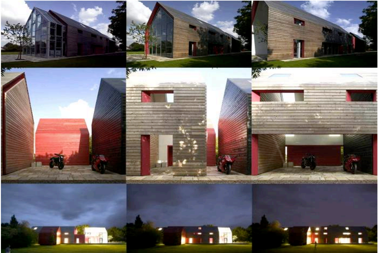
Figure 1.10- Sliding house: creating a movable sleeve the house is able to adapt along the seasons changes and benefit from the sun as a heating source. The covering sleeve, slides along tracks to allow the sun to penetrate through warming the building in cooler months. In warmer periods, the sleeve can be positioned to enclose the space, creating cooler conditions inside the space. The process takes around 6 minutes and it moves with a small motor. (Source: http://laurbana.com/blog/2013/02/07/sliding-house-de-drm-architects-la-casa-deslizante/ )
