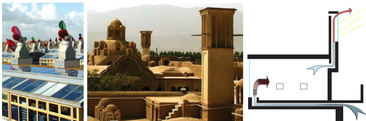
Figure 4.7- (Left and Right) New vs old and traditional, (Right) Wind Tunnel and chimney view for cooling in hot climates (Source: (Left) http://en.wikipedia.org/wiki/BedZED ; (Middle) http://wikitravel.org/en/Kashan ; (Right) Mafalda Melo Oliveira, 2014 based on (Velux Group , 2010))
